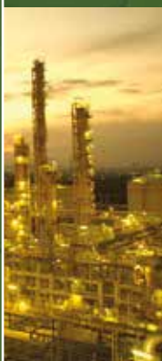
Petrochemical and Refinery
